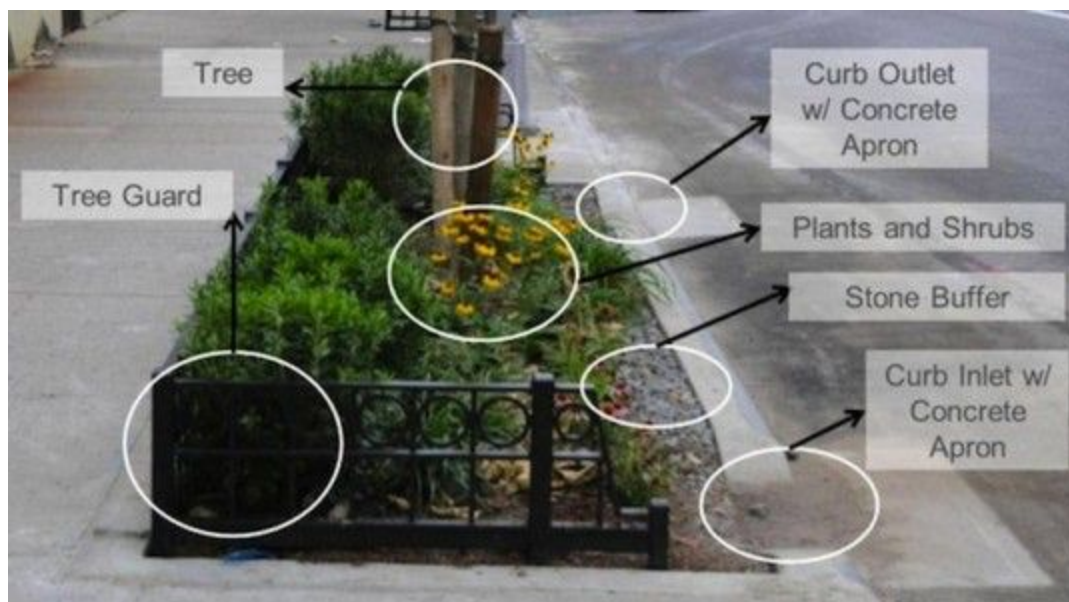
Figure 19: A example of a sidewalk garden design from the New York Department of Environmental Protection. You can see the use of flowering plants as well as trees and native shrubs (New York Department of Environmental Protection, 2018)
