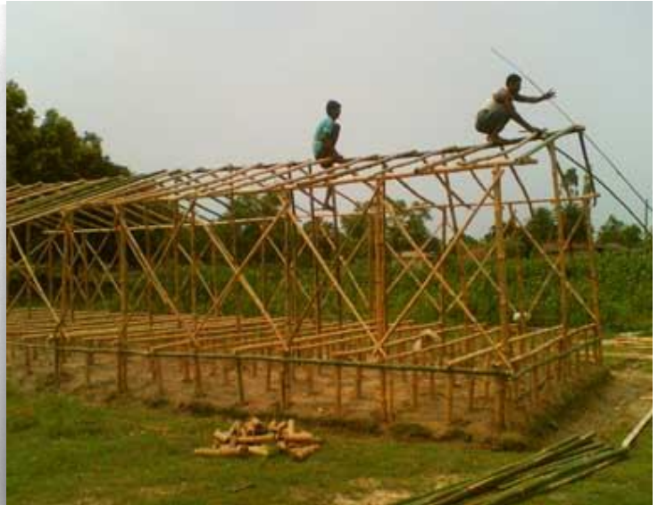
Figure 27 Bamboo house being built, showing cross bracing. (28)
