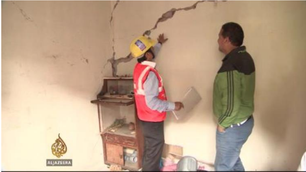
Figure 14 Interior of a damaged concrete building. Here, you can see clearly the direction in which the earthquake caused the crack to travel. (12)
