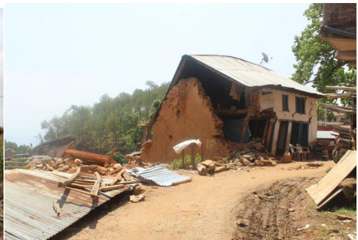
Figure 18 Adobe house after earthquake (23)
